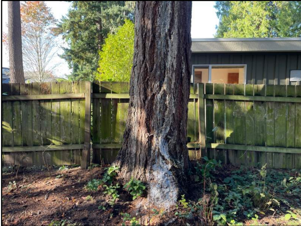
Photograph 4. Heavy pitch flow at the base of tree 593. This pitch is likely associated with an internal crack.
